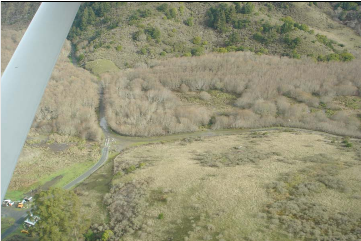
Figure 2. Aerial view of the second bridge crossing after high flows on January 28, 2008. Note ponded water at culvert locations and southern approach.
